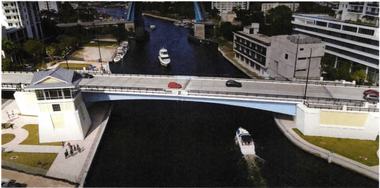
First Street Bridge
