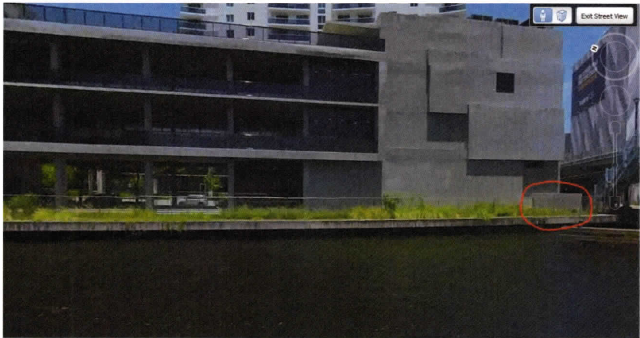
Small Stairway to be Removed
